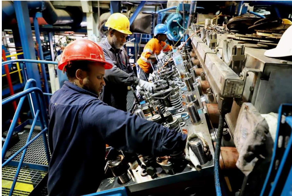
Figure 2: Overhaul at Lungga
