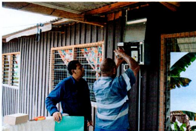
SP Technicians installing meters for a OBA recipient at Foxwood
