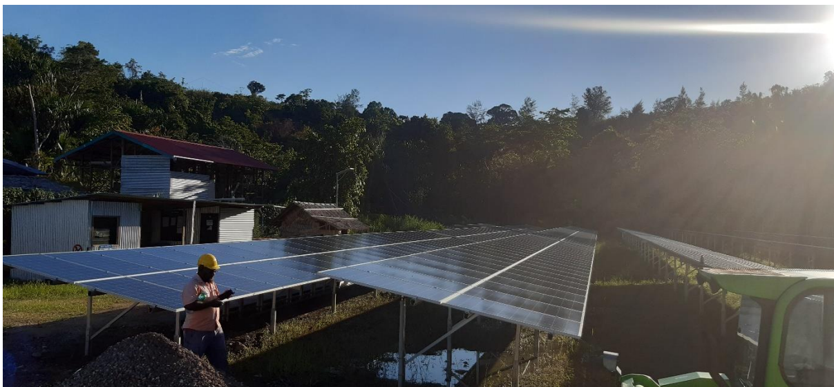
Figure 4. Tulagi solar farm- progress
