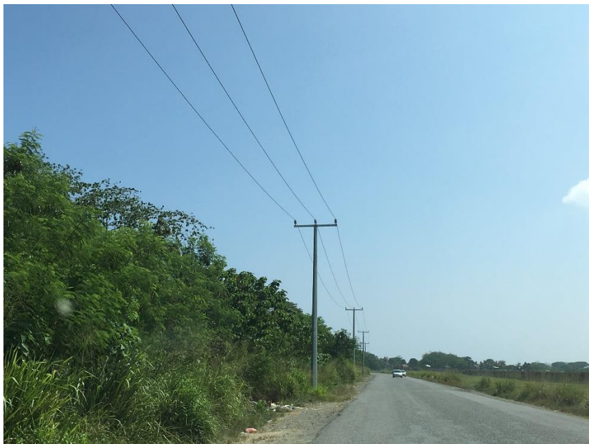
Figure 5. New Feeder 12 in Honiara
