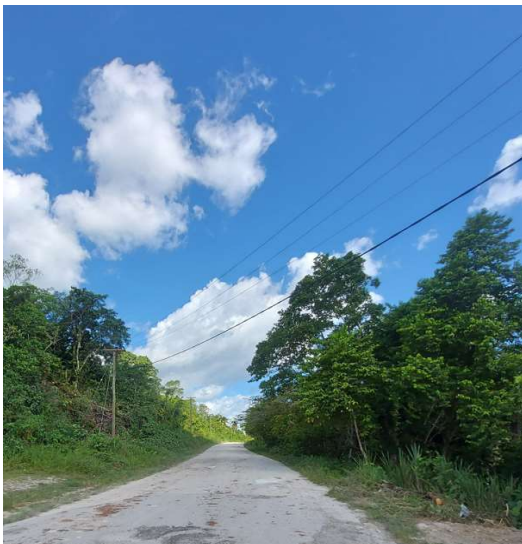
Figure 3. Network Extension at Kwainaketo, Malaita Province
